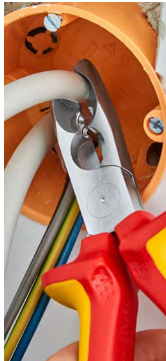
Stripping deep down in a flush-mounted junction box
